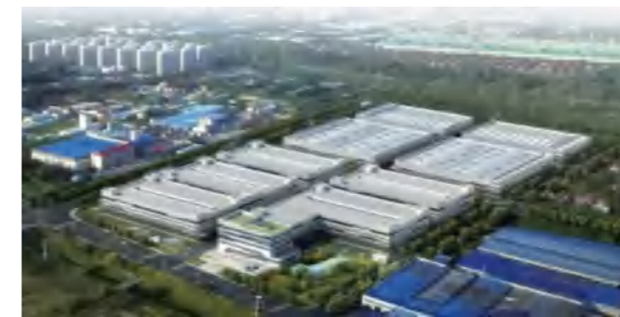
• Binzhou High-end Equipment Manufacturing Industrial Park
